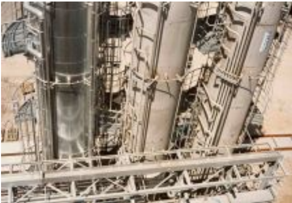
Refinery MIRO GmbH, Karlsruhe, Germany, March 1995 – Oct 1995 View image
